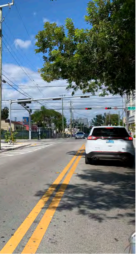
Location 1 - Striped out Shoulder
