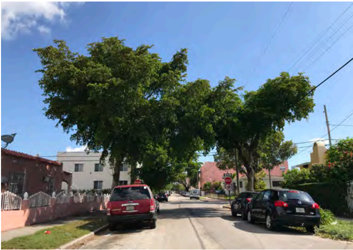
SW 5th Street - mature Black Olive trees ( Bucida buceras ) utility conflict on one side of the street.
