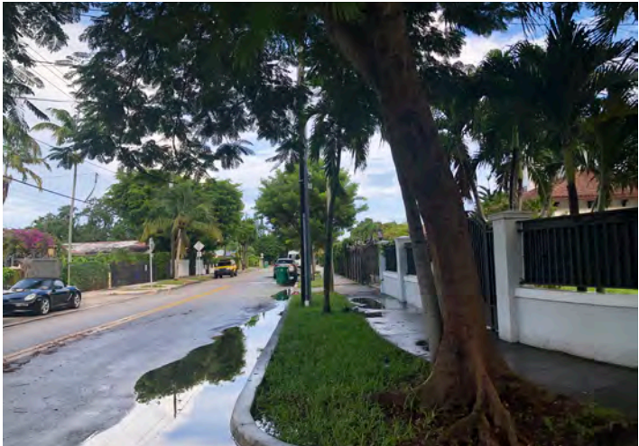
Flooded Swales at SW 21st Avenue & 24th Terrace
