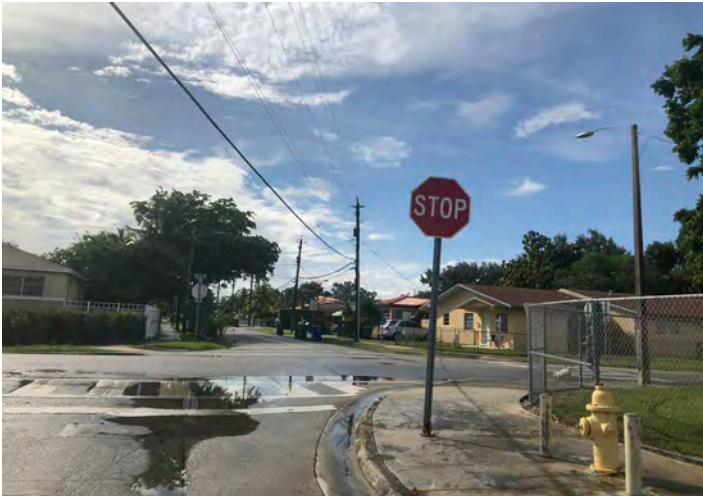
Flooded Swale at SW 14th Avenue & SW 20th Street
