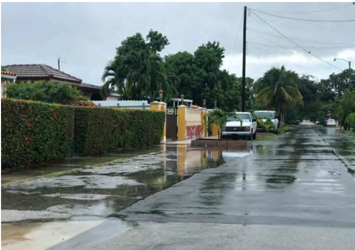
Flooded Swale SW 12th Street
