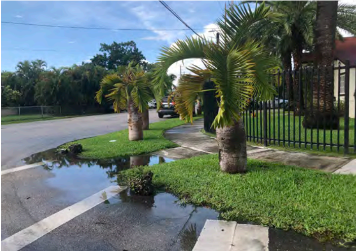
Flooded Swales at SW 16th Avenue & SW 21st Street
