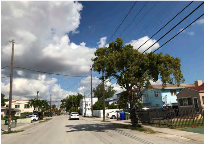
SW 19th Avenue - Black Olive ( Bucida buceras ) conflicting with power lines.
