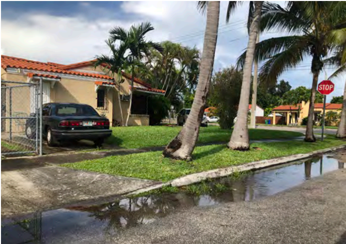
Flooded Swales at SW 22nd Avenue & 24th Street
