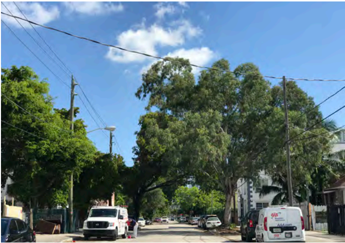
SW 2nd Street - Eucalyptus ( spp. ) on right and Mahogany ( Swietenia mahagoni ) on left both conflicting with utility lines
