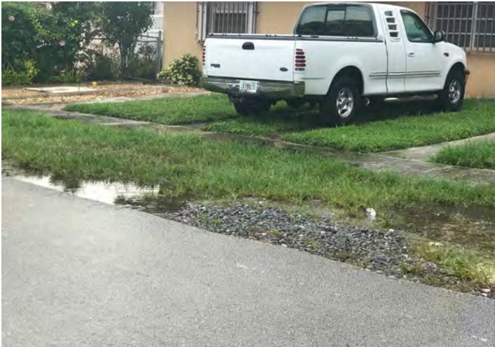
Flooded Swale at SW 13th Terrace
