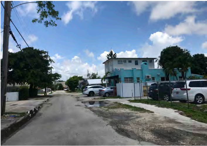
Standing water on compacted dirt swale at 4th street and 21st avenue
