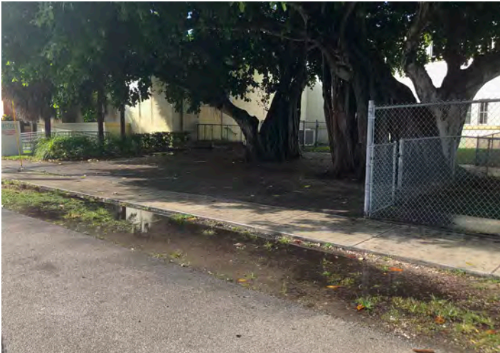
Flooded swale at SW 13th Avenue & SW 20th Street
