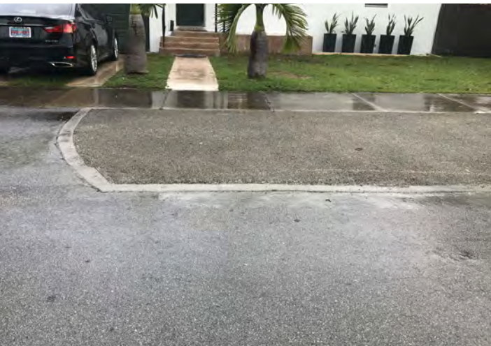
Porous Asphalt installation on SW 19th Terrace - seen in several locations in this neighborhood
