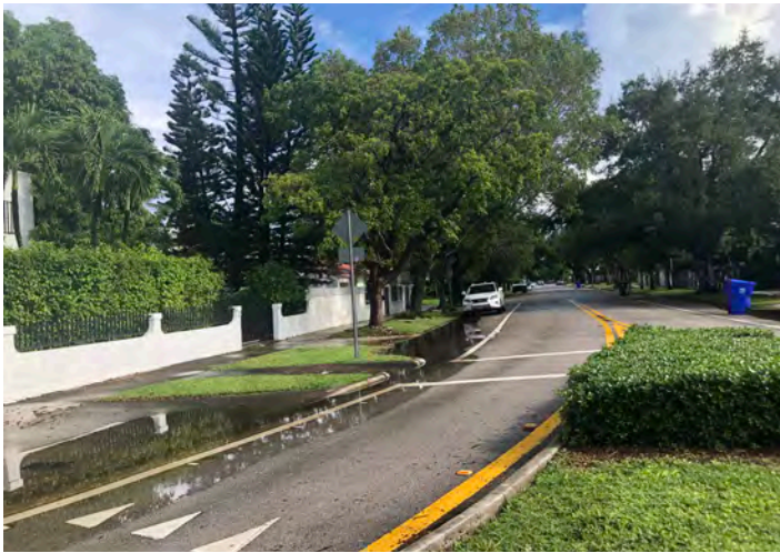
Flooded Driveways, on-street parking and crosswalk overflowing onto swale at SW 28th Road
