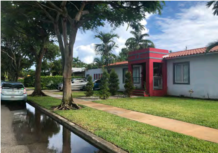
Flooded Swale at SW 21st Avenue & SW 23rd Street
