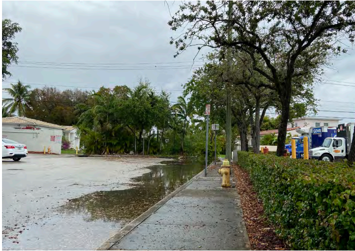
Flooded on-street parking on SW 33rd Avenue
