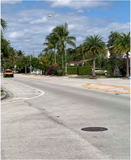
Location 6 - Striped out Shoulder
