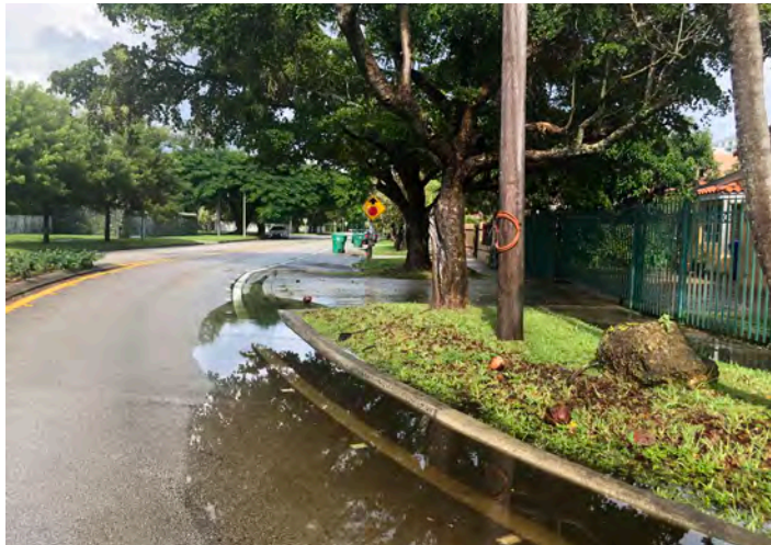
Flooding overflowing onto swale at SW 29th Road
