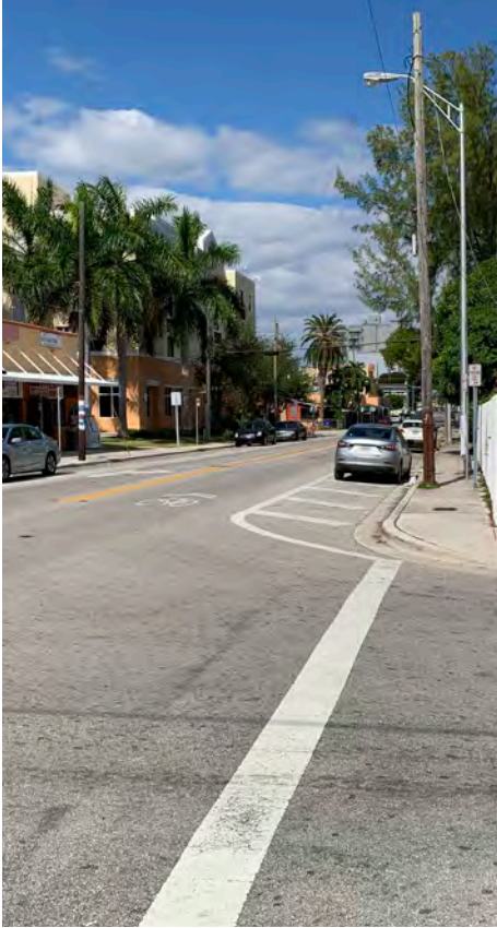
Location 5 - Striped out Shoulder
