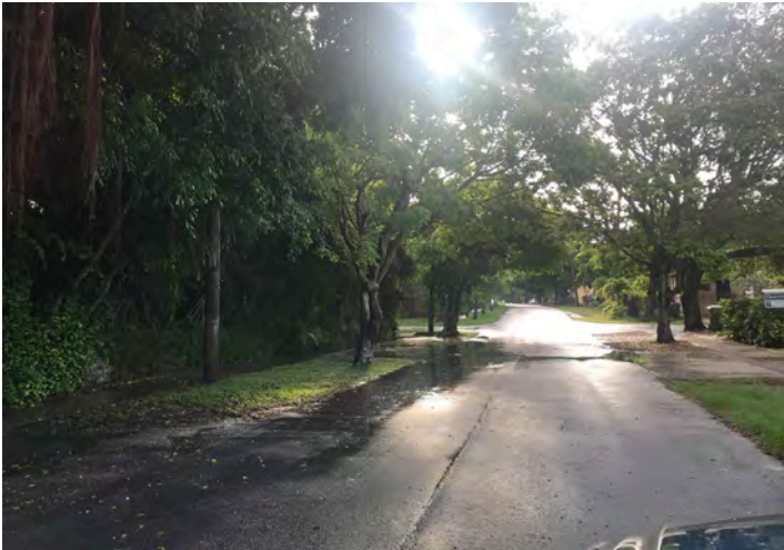
Flooded Swale at SW 29th St near SW 33rd Ct.
