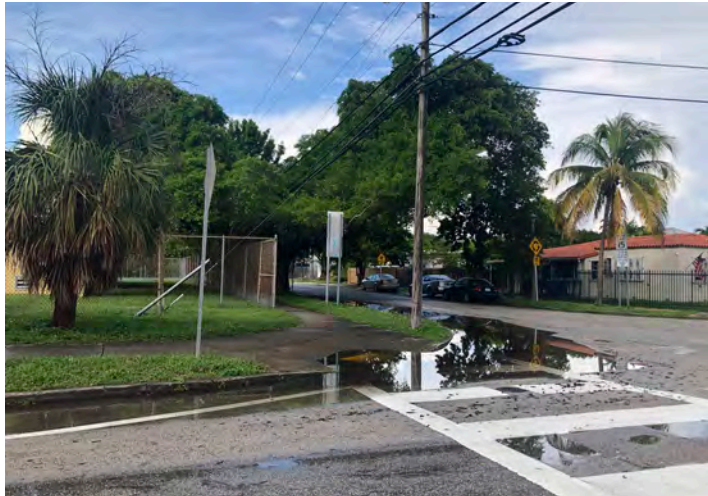
Flooded Swale at SW 24th Street & 26th Terrace
