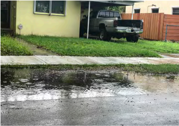
Flooded Swale at SW 11th Street
