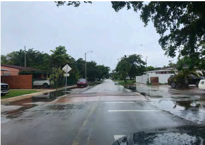
Flooded Swales at SW 11th Street
