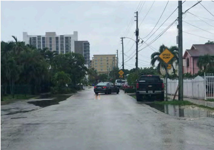
Flooded Swale at SW 15th Street
