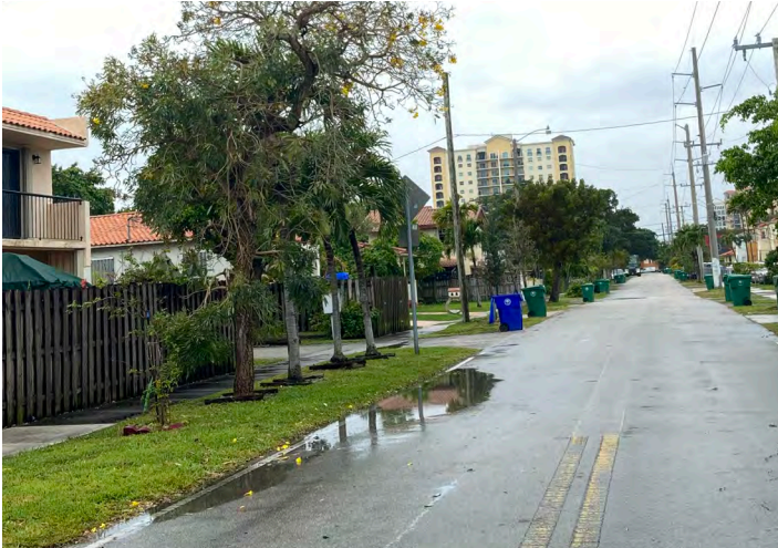
Flooding along street at SW 16 Terrace and Coral Gate Drive
