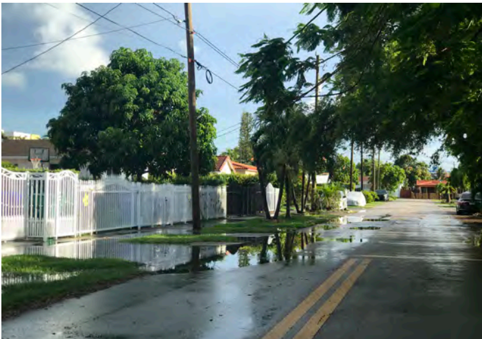
Flooded Swales at SW 27th Street near SW 33rd Ct
