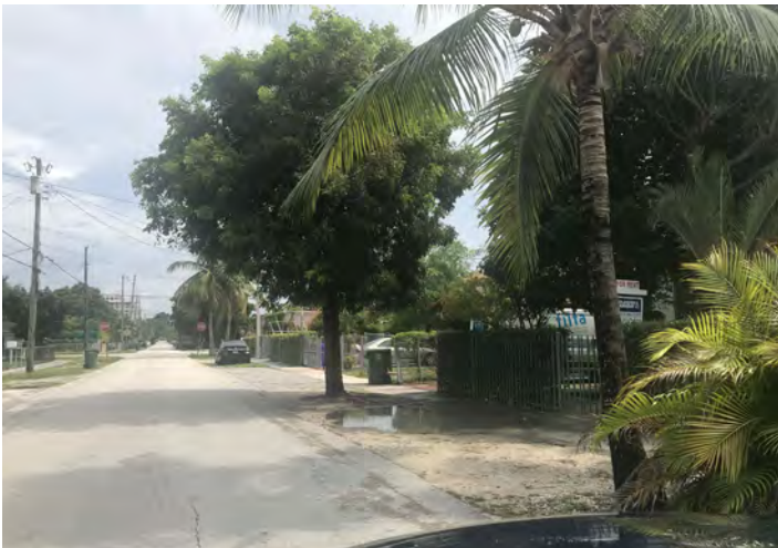
Flooded Swale at SW 11th Street
