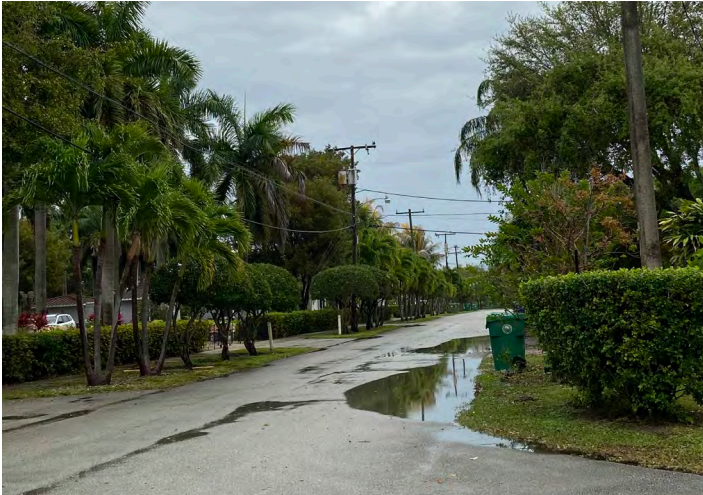
Flooding along street at SW 17th Street and SW 35th Court
