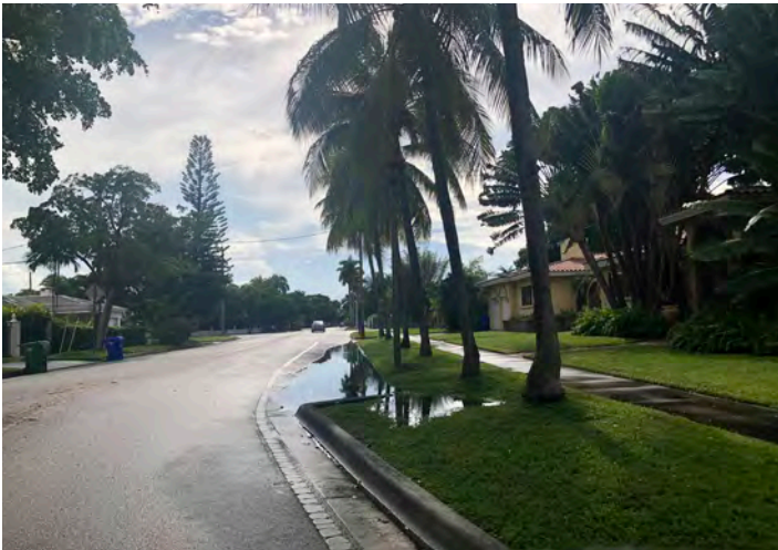
Flooded on-street parking and portion of swale at SW 7th Ave.
