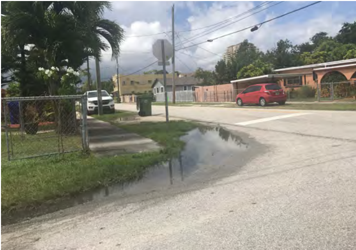
Flooded Swale at SW 12th Street
