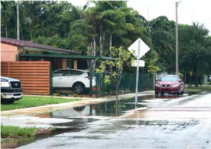
Flooded swale with tree at SW 11th Street
