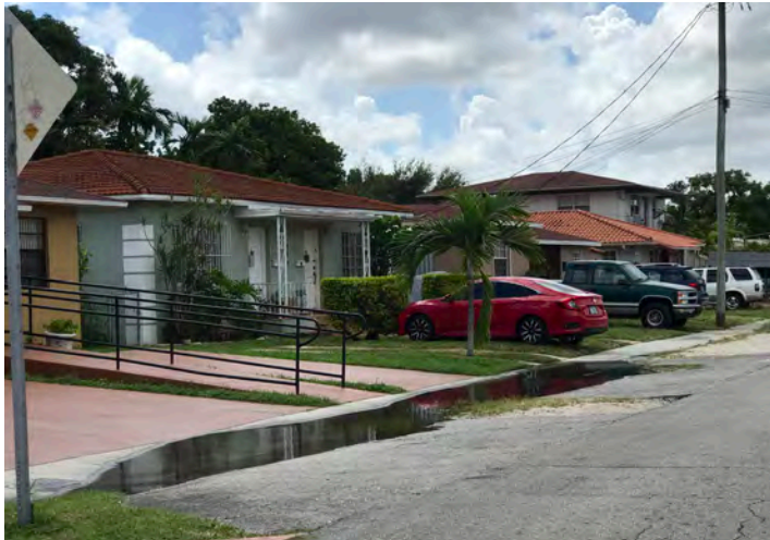
Flooded Swale at SW 2nd Street
