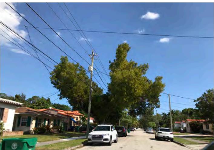
SW 16th Avenue - Mature tree being Y-cut for utility lines
