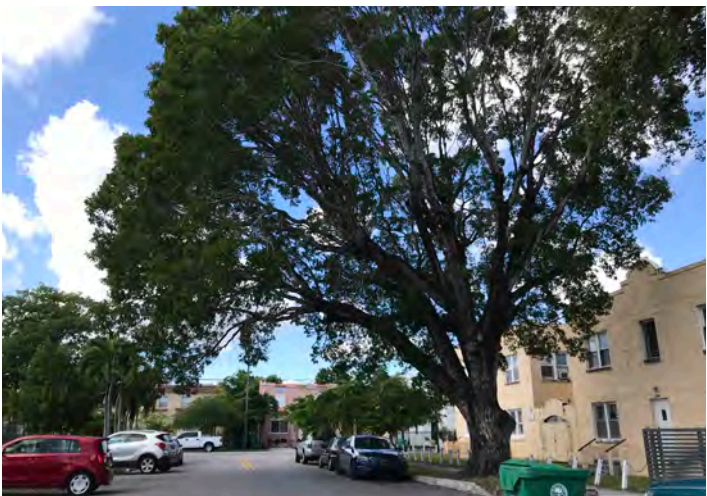
SW 11th Street near 19th Avenue - Mahogany ( Swietenia mahagoni ) with constricted roots lifting curb and sidewalk
