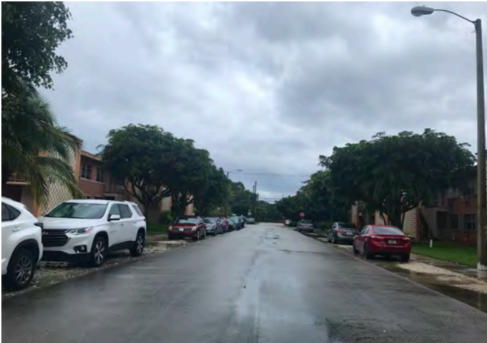
Flooded Swales at SW 9th Terrace
