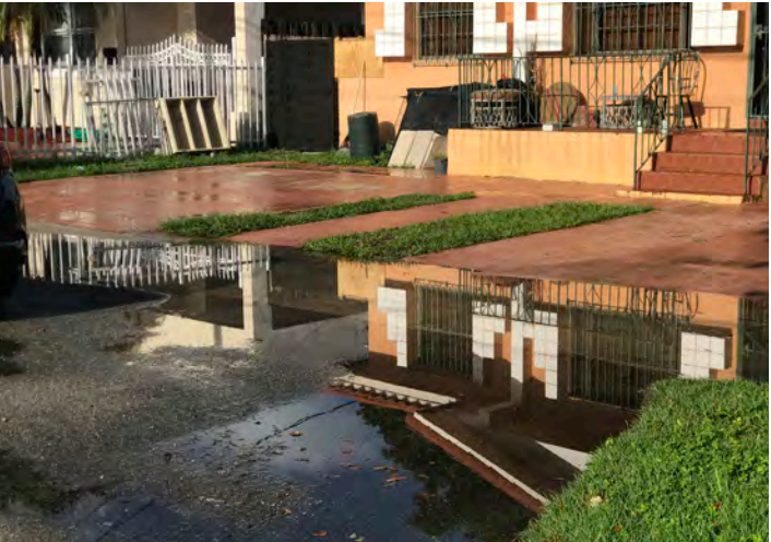
Flooded Swale at SW 34th Ave near SW 28th St.
