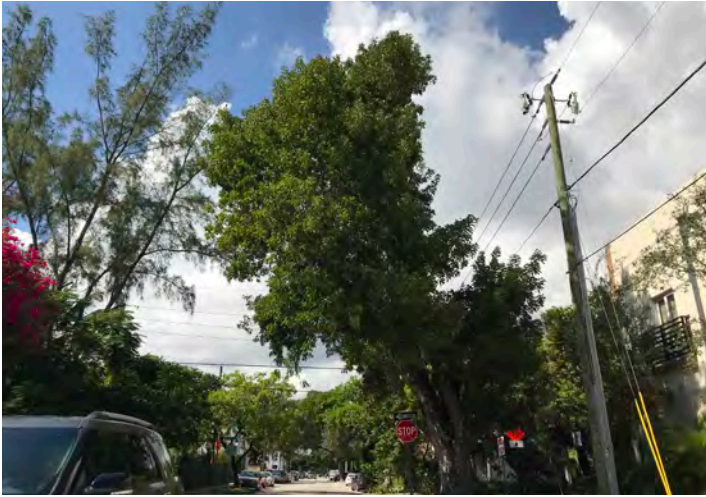
SW 2nd Street - Mahogany ( Swietenia mahagoni ) lopsided with utility line conflict
