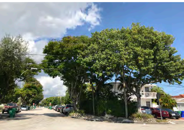
SW 12th Street - Mature trees interfering with utility lines
