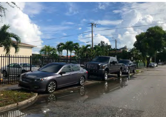
Flooded valley gutter at SW 10th Street and SW 7th Avenue
