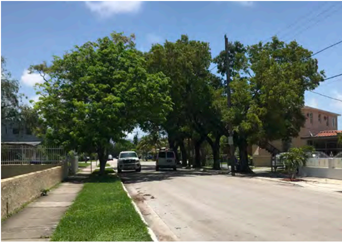
SW 4th Street and Beacom Boulevard - Golden Shower ( Cassia fistula ) on left and Mahogany ( Swietenia mahagoni ) on right conflicting with utility lines
