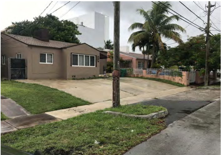
Completely paved frontage, showing elevation change typical of houses in this area - porous asphalt in front
