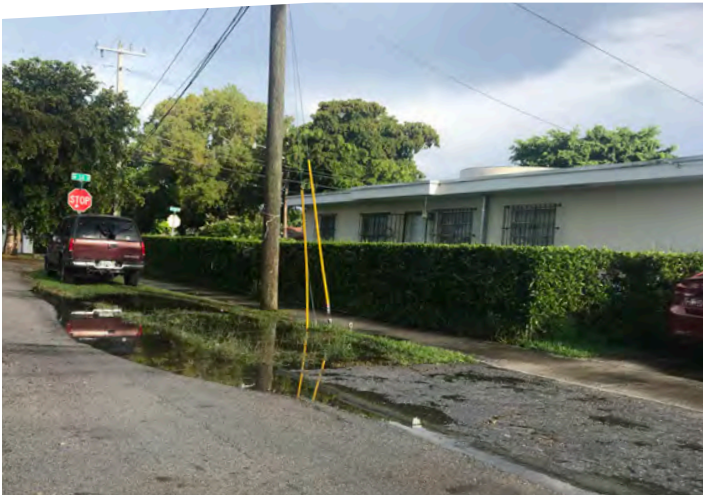
Flooded Swales at SW 36th Avenue
