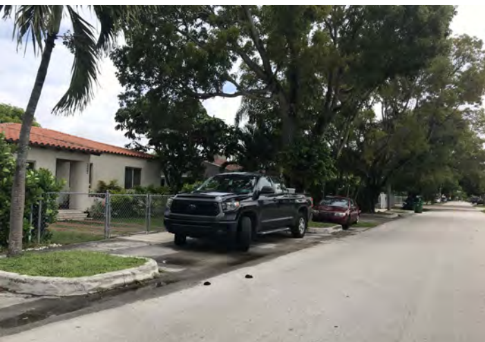
Curbs on SW 20th Street - appear to be only in some places
