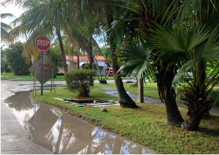
Flooded Swale at SW 21st Avenue & SW 25th Terrace
