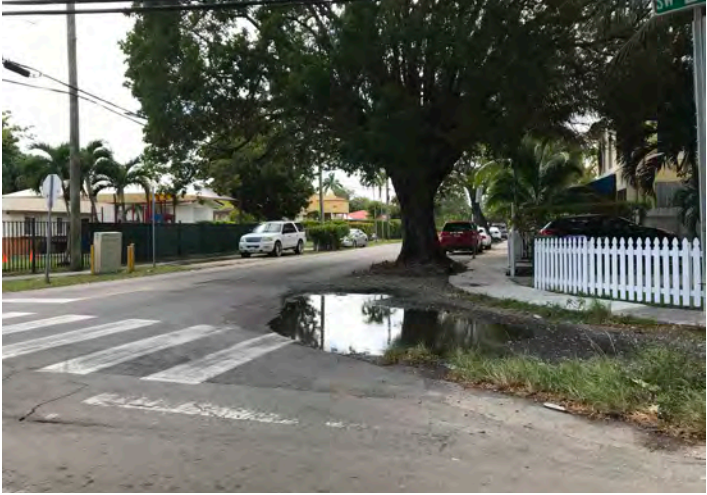
Flooded Swale at SW 29th Avenue and SW 6th Street
