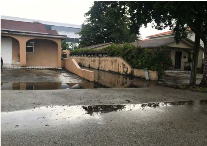
House with completely paved frontage and standing water in driveway on SW 21st Street
