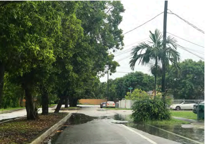
Flooded Road & Swale at SW 33rd Avenue
