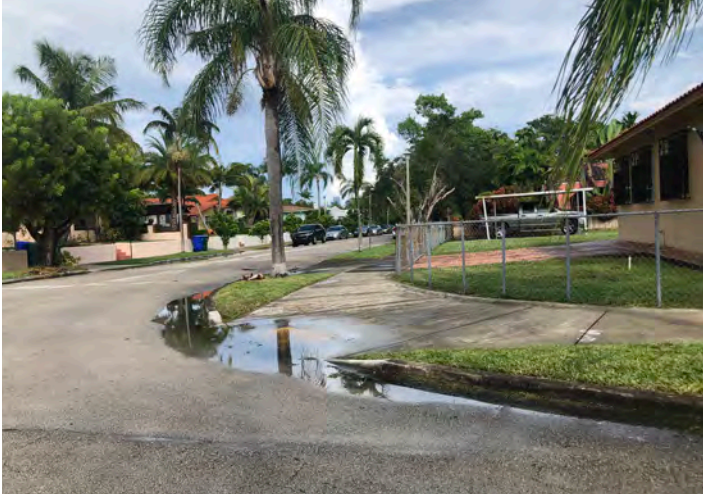
Flooded Swales at SW 24th Avenue & SW 23rd Terrace
