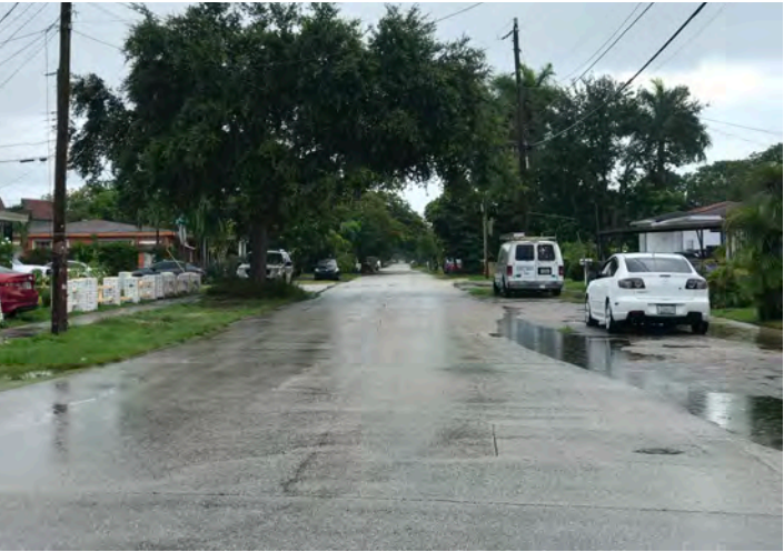
Flooded swale at SW 13th Street
