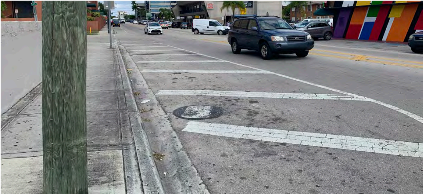
Figure 2-2: Location 2 - Painted Shoulder
