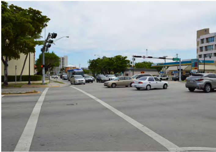
Figure 18: SW 27th Avenue
