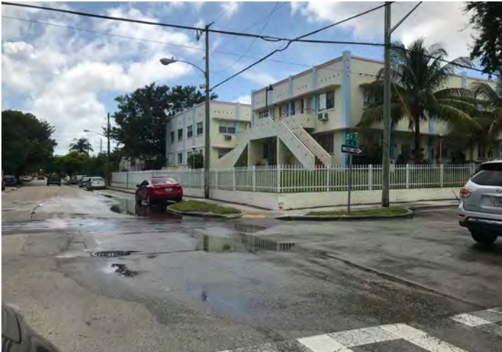
Backed up storm drain at SW 4th Street and SW 6th Avenue
