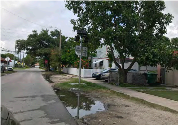
Flooded Swales at SW 29th Avenue
