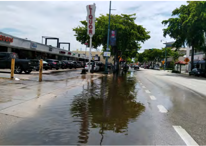
Backed up storm drain at SW 8th Street and SW 9th Avenue
