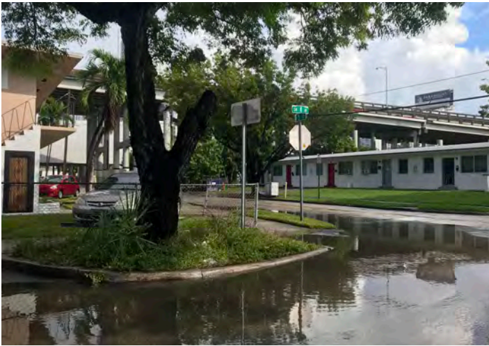
Backed up storm drain at SW 5th Street and SW 4th Avenue
