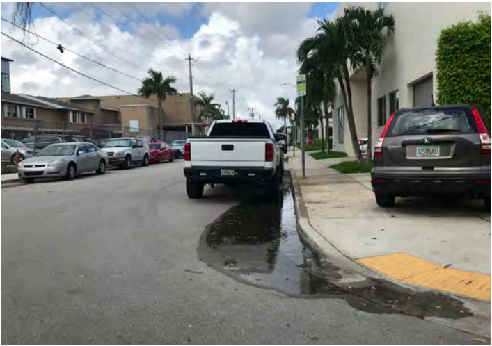
Flooded street side at SW 9th Street and SW 7th Avenue
